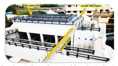
Fig.4: Ozonation System - Pre-Aeration & Ozone Reaction Chamber and Treated Effluent Storage Tank
