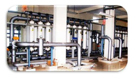
Fig.3: Ultra-filtration (UF) system
