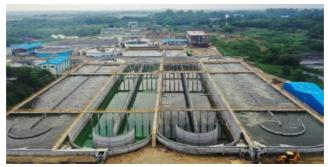
Figure 3: 20 mld CETP in Jajmau is at advanced stage of construction (Photo: Sajid Hussain)
